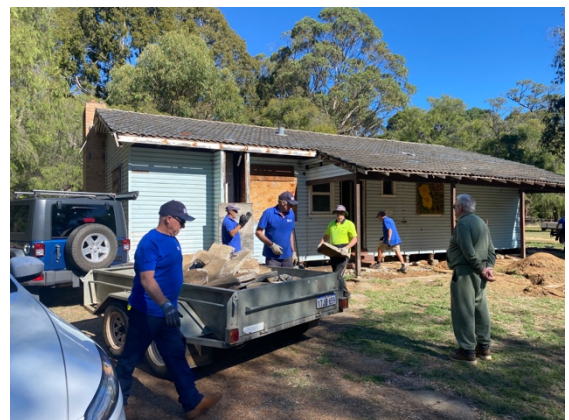
Photo: The Blue House renovation
