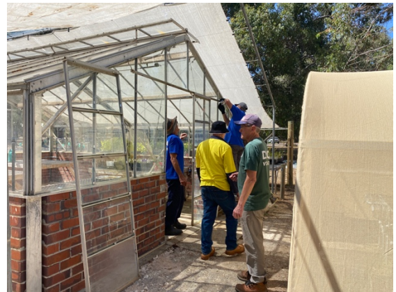
Photo: Glass house renovation
