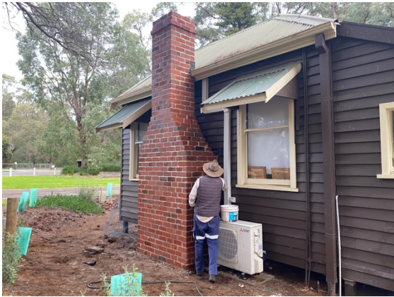
Photo: New District office chimney
