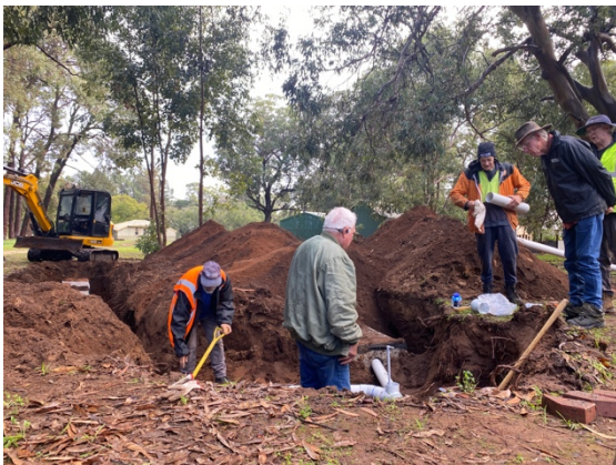
Photo: New leach-drain installation
