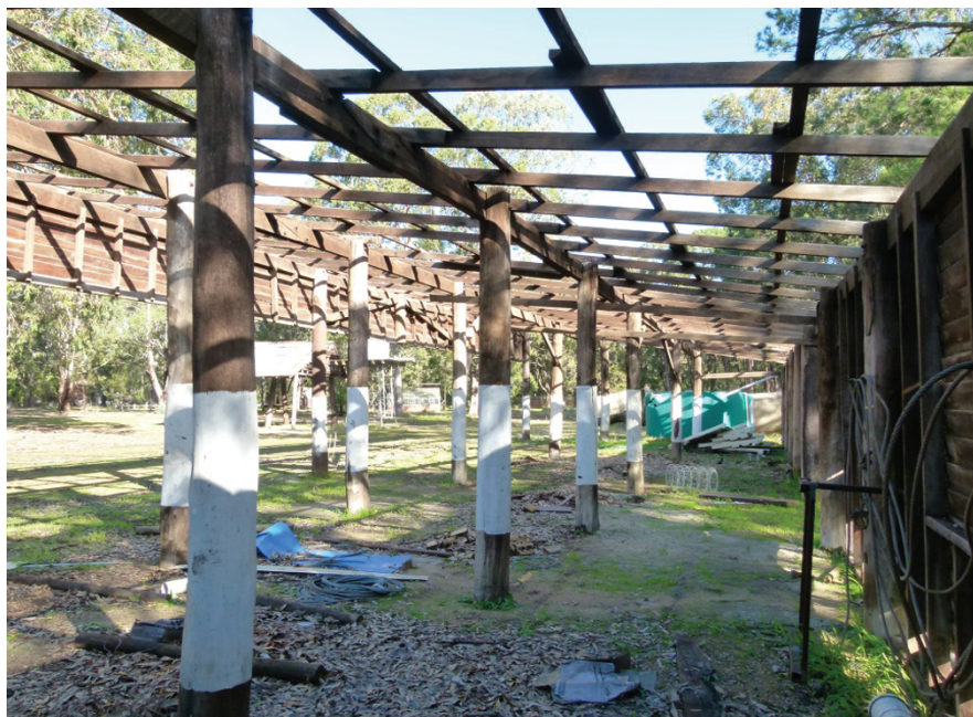
Figure 7. Truck bay shed before restoration. The asbestos roof has been removed, and some timber structural members and weather boards replaced. Photo: Des Donnelly.
