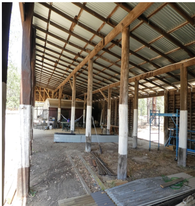
Figure 8. Truck bay shed after restoration. The building has been straightened up, a new 285 m 2 zinc alum roof fitted together with a 110,000 L rainwater tank which provides potable water to the Ludlow Settlement. This work was carried out by Department of Corrections, Bunbury, Section 95 work release parolees, and the Ludlow Tuart Forest Restoration Group community volunteers. The project was funded by a City of Busselton community grant of $19,000. Photo: Des Donnelly.
